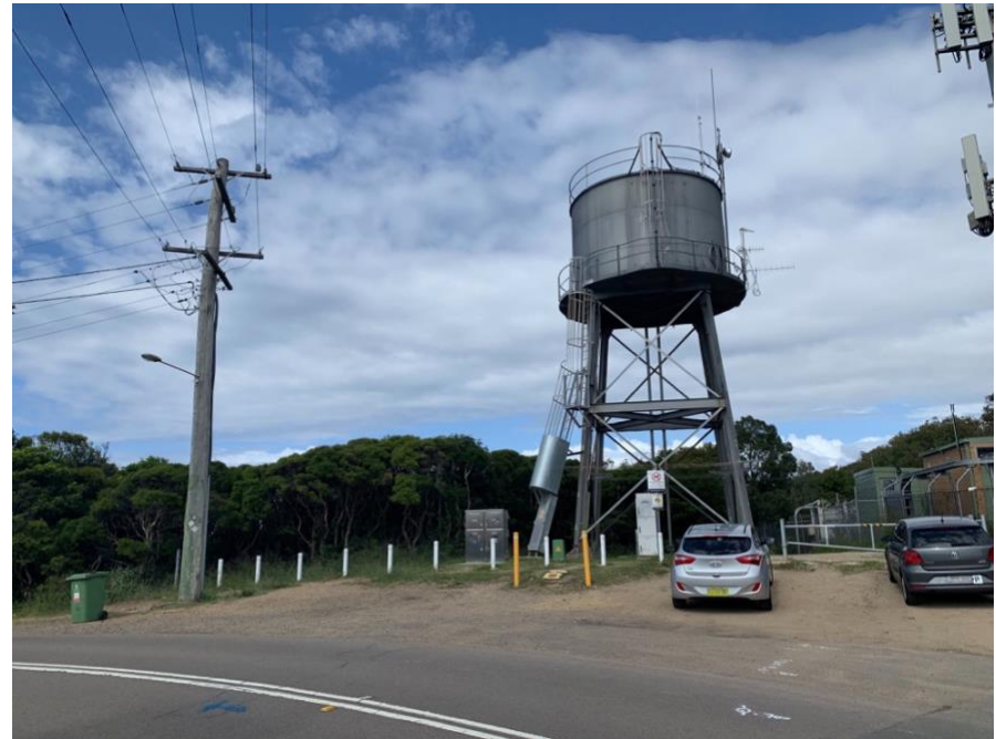
Plate 5-4 view of site from opposite side of Hickson Street looking south
