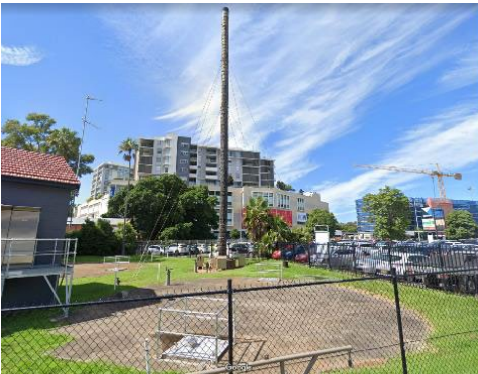
Photo 6-1. Nexsting NW1 WWPS wooden vent stack against high-rise buildings (source: Google, 2022)
