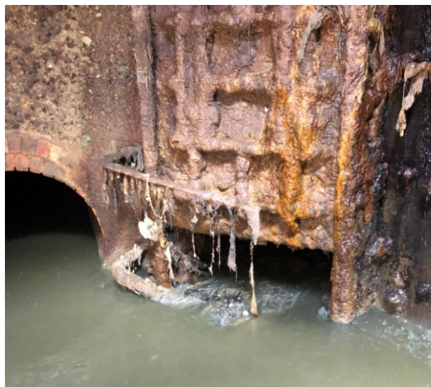
Photo 2-2: North-western penstock corrosion
