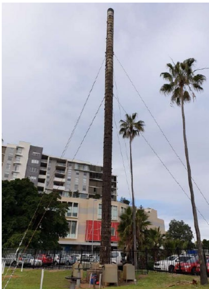
Photo 2-3: Existing Wooden Vent Stack
