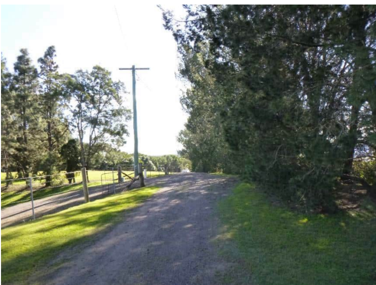
Photo 5-2 Access Road to existing reservoir
