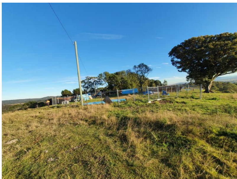
Photo 3-2 The location of the new reservoir, photo taken from the existing reservoir facing north west
