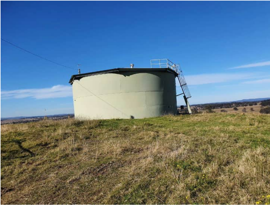
Photo 2-2 The existing reservoir
