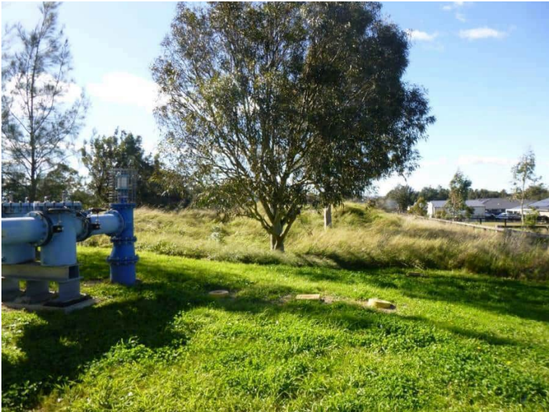
Photo 5-7 Buried infrastructure at Lochinvar WPS, view to the north east
