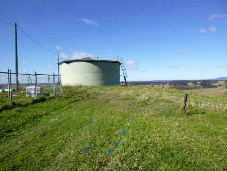
Photo 5-3 Lochinvar Reservoir, view to the southeast
