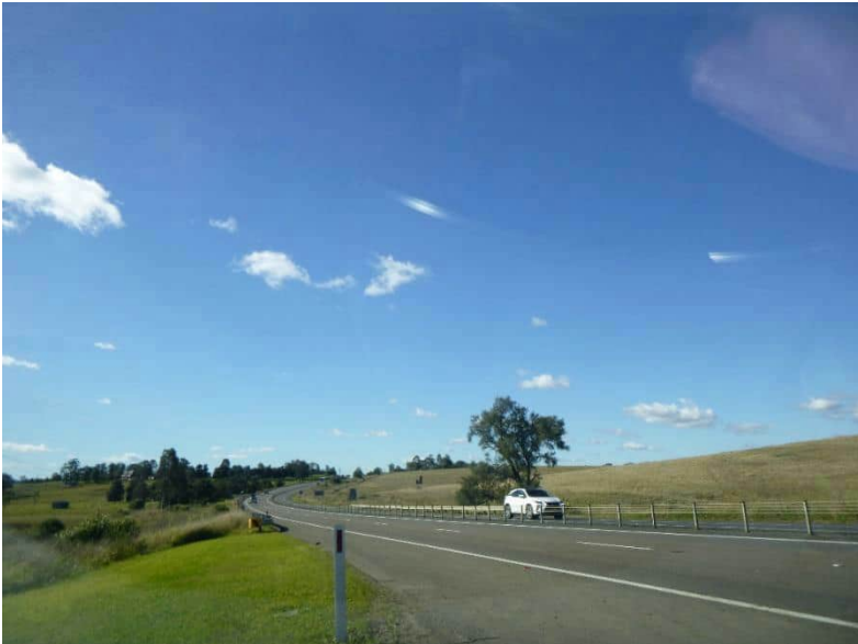
Photo 5-5 New England Highway over culvert, view to the southeast
