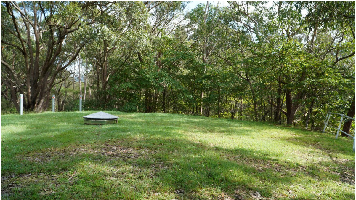
Plate 4. View north-west across the top of the underground reservoir, showing the octagonal cast-iron vent
