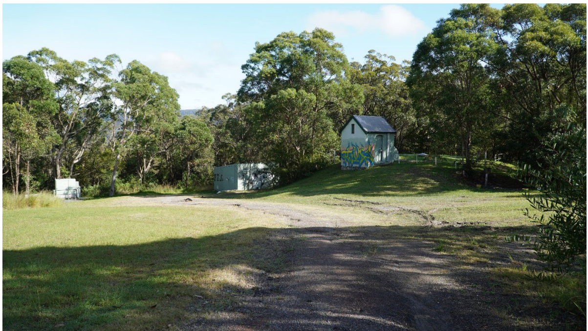
Plate 1. View north-west towards valve house and reservoir (building to the right of frame overlying the reservoir mound), the pumping station building (centre of frame) and the modern pumping station structure (left of frame).
