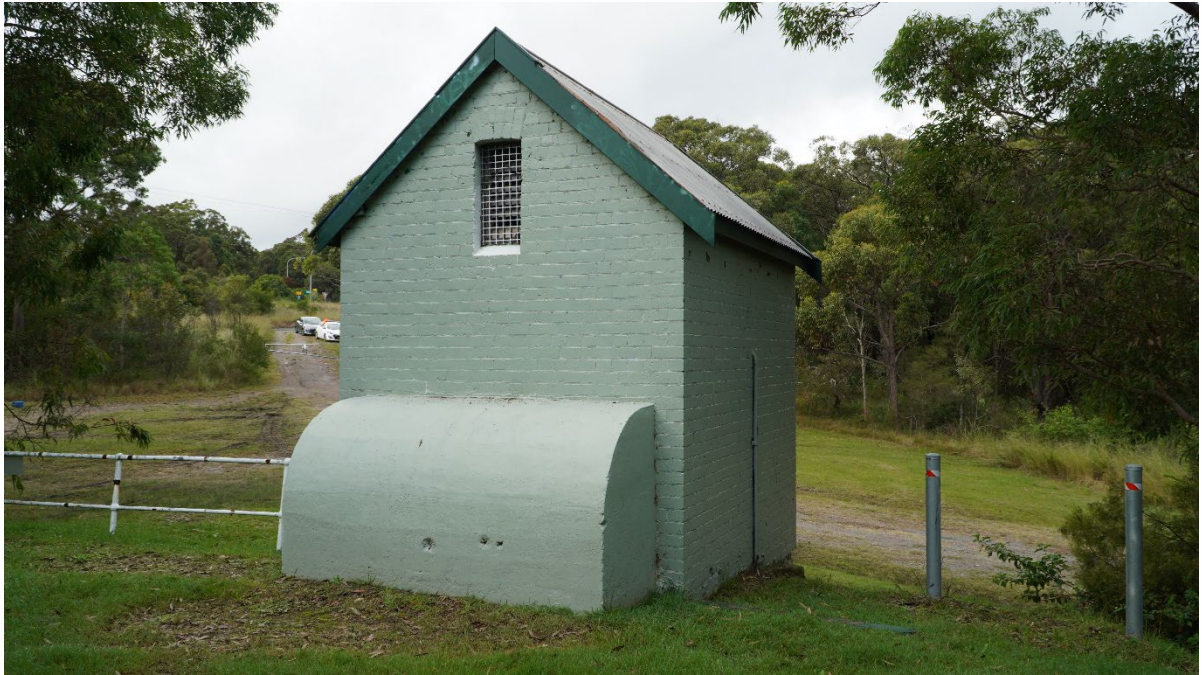
Plate 7. View of the southern side of the valve house (onto of the reservoir) facing south-east.
