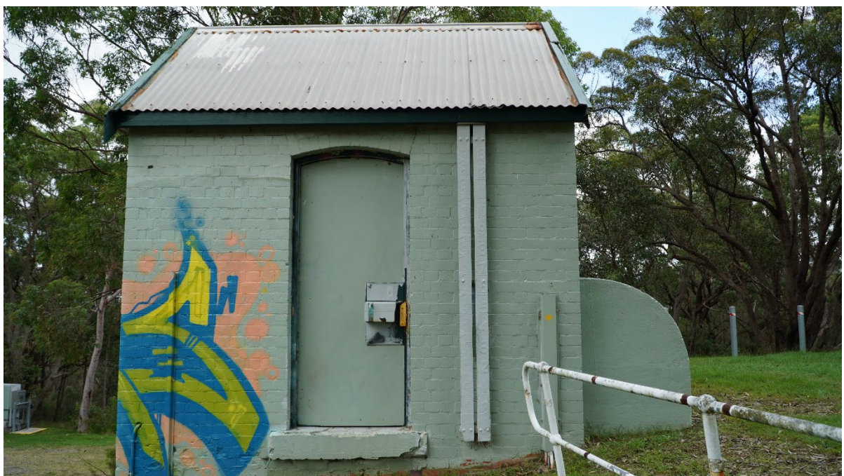
Plate 6. Eastern side of the valve house (facing west), showing entrance.
