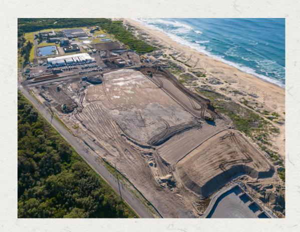
Work is powering ahead at our Belmont Desalination Plant site. Piling is continuing in the next few weeks so that work can soon begin on the onshore intake shaft excavation.
