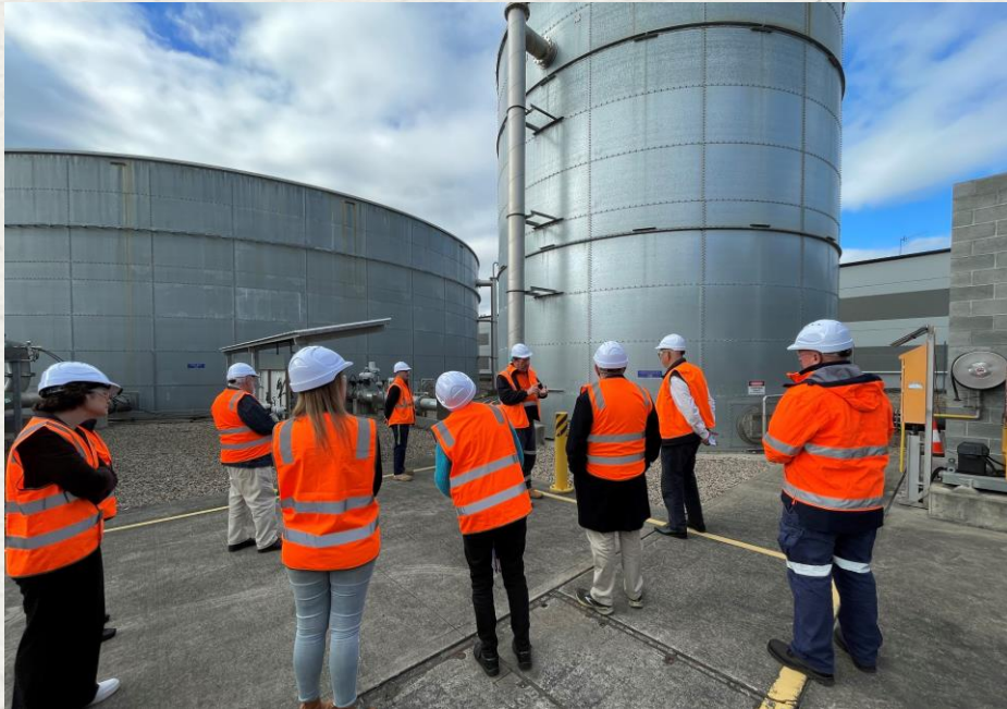
CCAG's site visit to the coNEXA Advanced Water Treatment Plant, June 2024.
