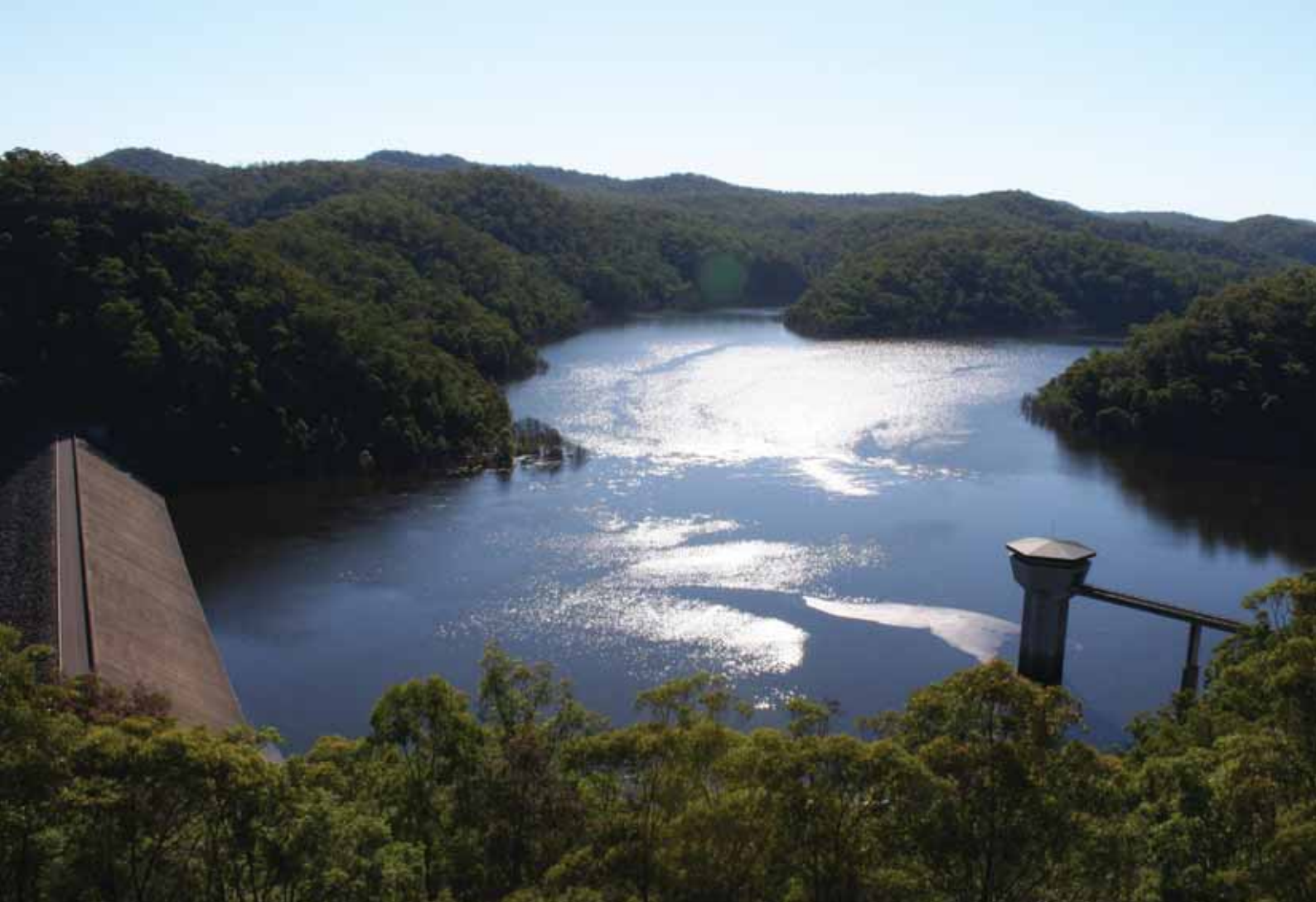
Mangrove Creek Dam
